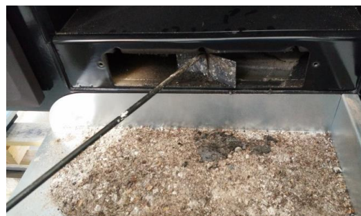
Figure No.20 - Accesses via which to clean the flue socket.
